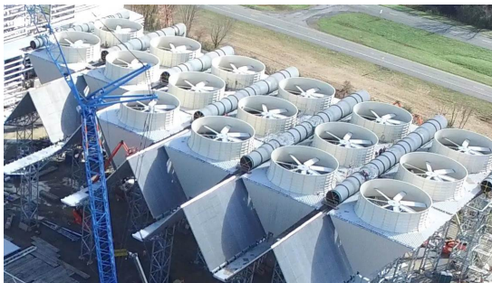
Figure: Induced draught air-cooled condensers (ACCs)
