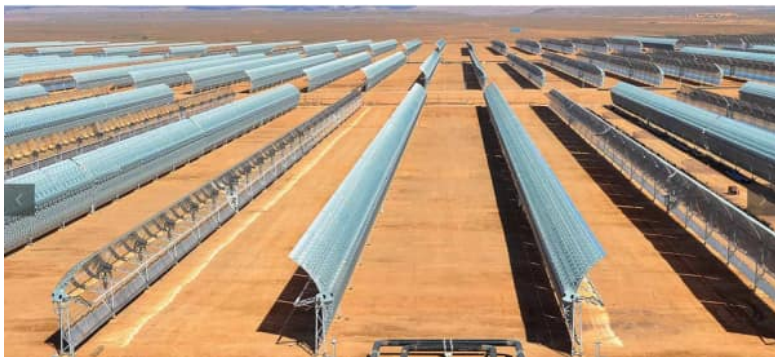
Figure: Kathu Solar Park
